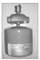
**Expansion Tank and Air Scoop:** The expansion tank and air scoop assembly is used to compensate for the expansion and contraction of liquid solution in the system. The air scoop eliminates air entrained in the liquid solution.
